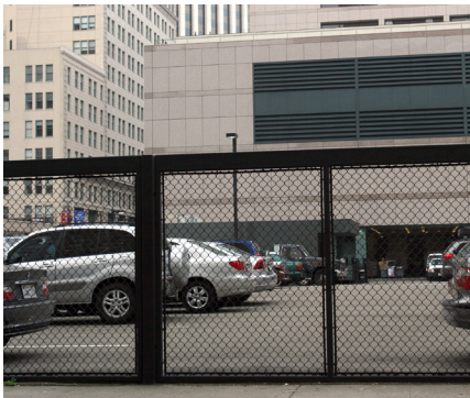
Federal Reserve Bank, 101 Market Street
