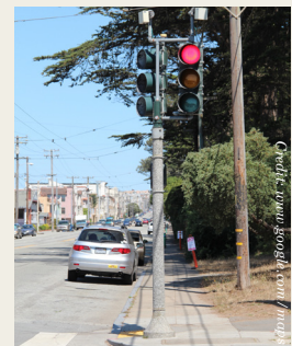
No sidewalk lighting
