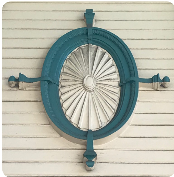
A Victorian ornamental detail found on the corridor.
