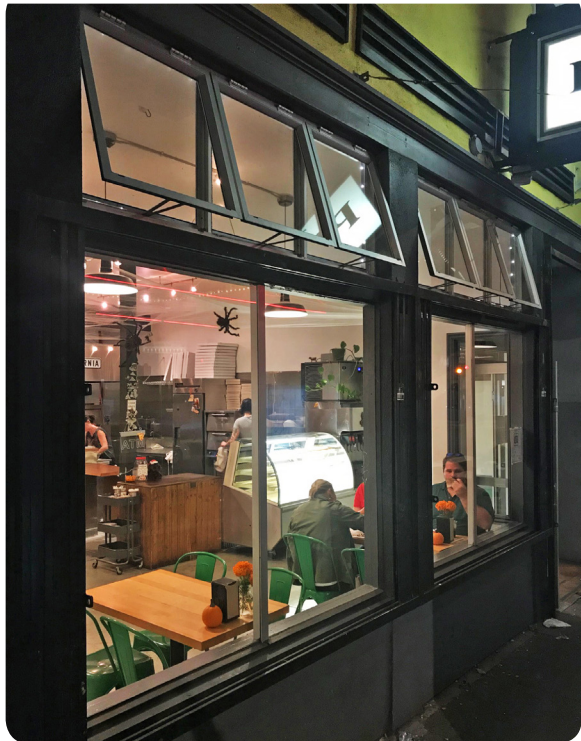
Operable transom windows address the pedestrian.
