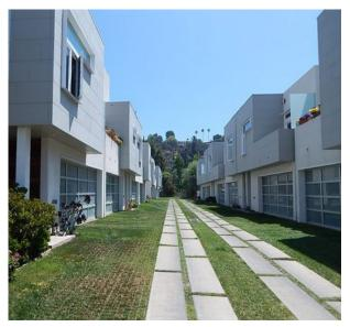
Permeable and vehicular rated paving is used to maximize pervious surface for stormwater management
