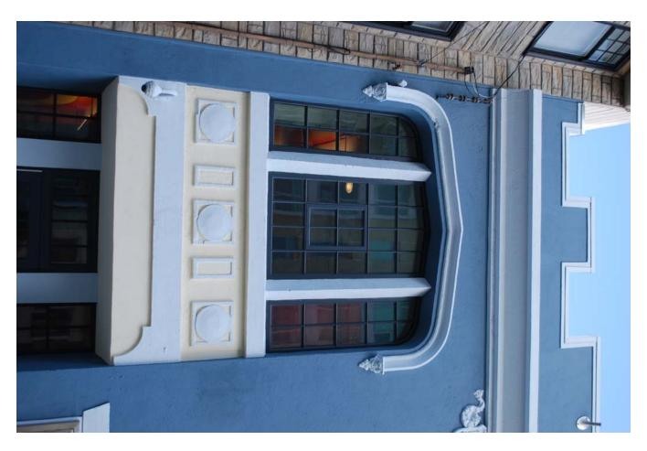
Window and cornice detail, showing new window sash that is virtually identical to the original. The parapet, cornice, drip molding, mullions, paneled spandrel, and lintel over the first story opening (with curved corners) are all original. The treatment of the other two bays is the same. Photo: October 2009.
