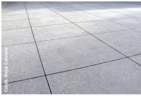
Enhanced cast-in-place concrete with saw-cut joints.
