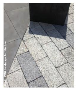
PERMEABLE CONCRETE UNIT PAVERS
