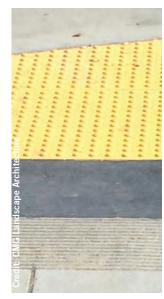
DETECTABLE SURFACE PAVING: SF PUBLIC WORKS STANDARD
