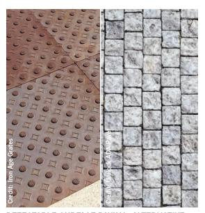
**DETECTABLE SURFACE PAVING: ALTERNATIVE**
