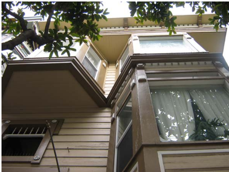
Detail showing upper portion of main façade. Source: Page and Turnbull
