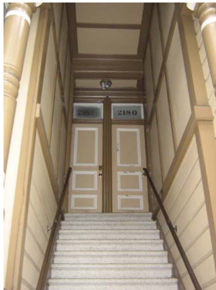
Detail of residential entrances on second story. Source: Page and Turnbull
