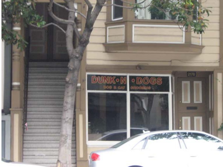
Detail of first story storefront. Source: Page and Turnbull
