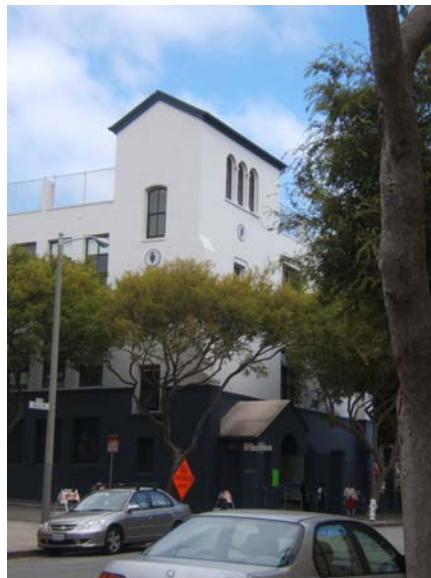
Southwest corner of building, showing tower and secondary entry. Source: Page and Turnbull
