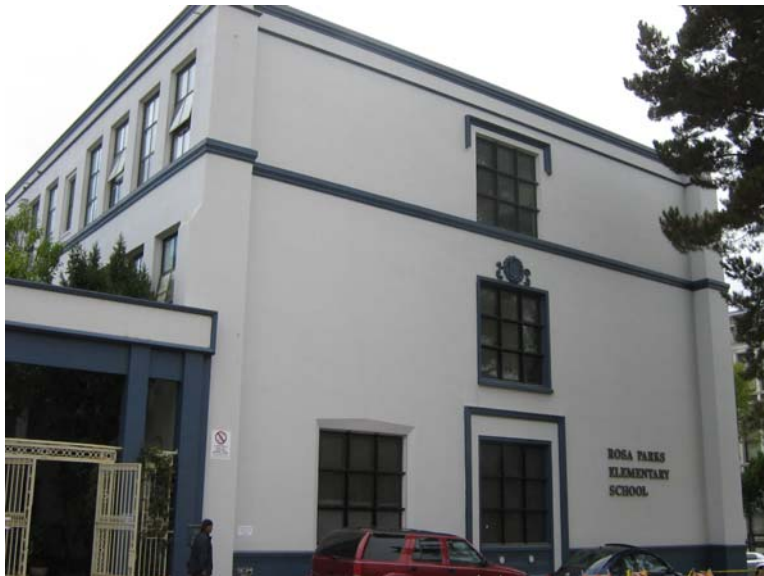
View of north façade of main building, looking southwest. Source: Page and Turnbull
