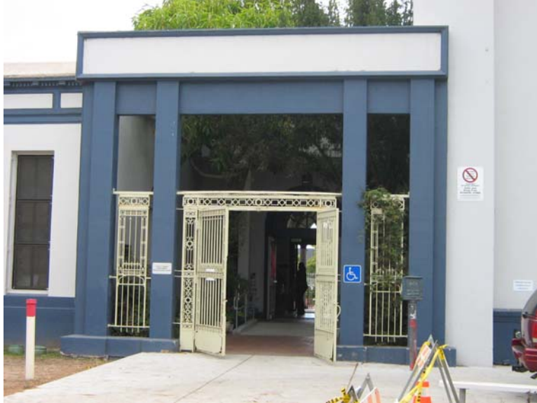
Detail of primary entrance into school complex. Source: Page and Turnbull
