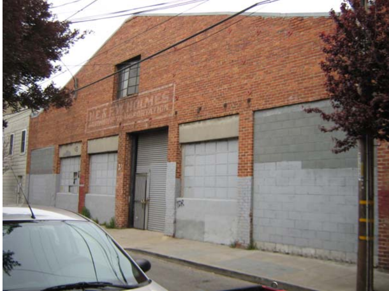
View of rear (west) façade. Source: Page and Turnbull
