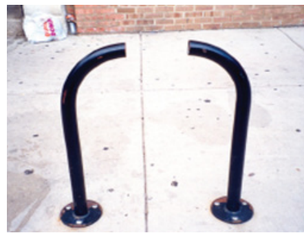
Unacceptable These bicycle racks either provide only one point of support for bicycles, are constructed with round tubed material which makes them prone to cutting, or do not allow locking a frame and wheel directly to the rack with a U-lock.
